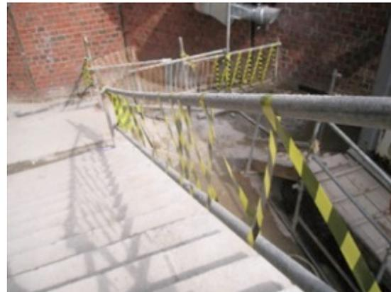
Figure 2 Handrails at open edges of stairway
