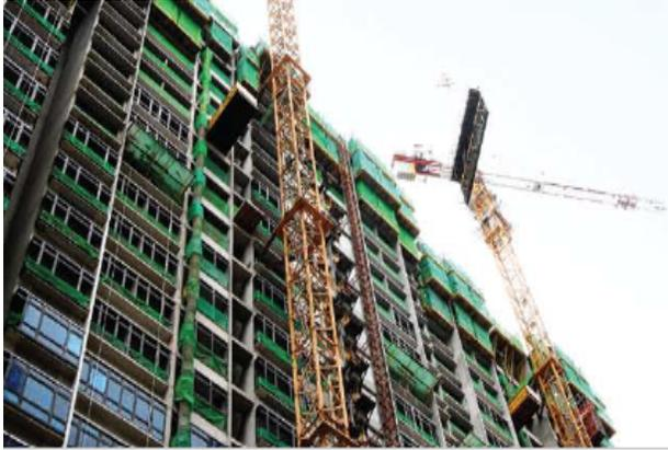
Figure 5 Example of netting for high rise construction
