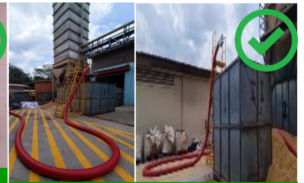
Engineering control with a proper platform
