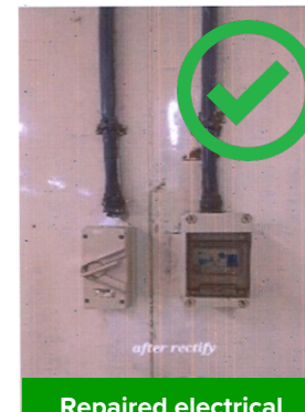
Repaired electrical installation
